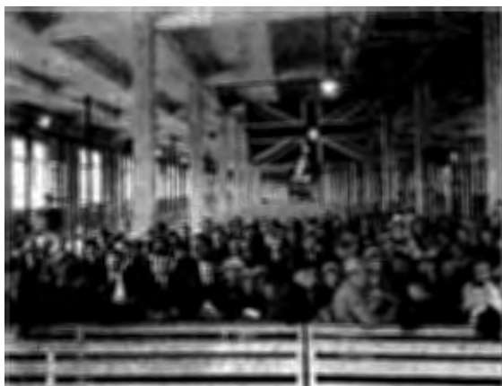
Interior of Immigration Hall, Louise Embankment, Port of Québec, c 1900. Credit: Library and Archives Canada, a048697
