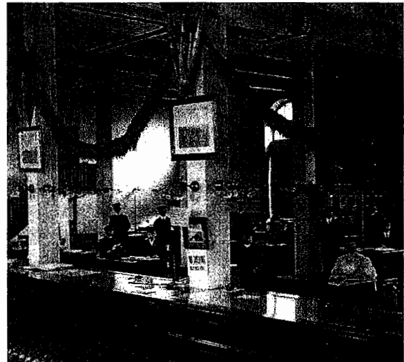
Fig. 6 Dominion Immigration Building – interior, Library and Archives Canada, C075993.
