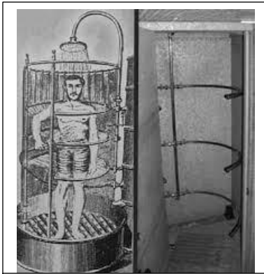
Shower System in Disinfection Building (Parks Canada)
